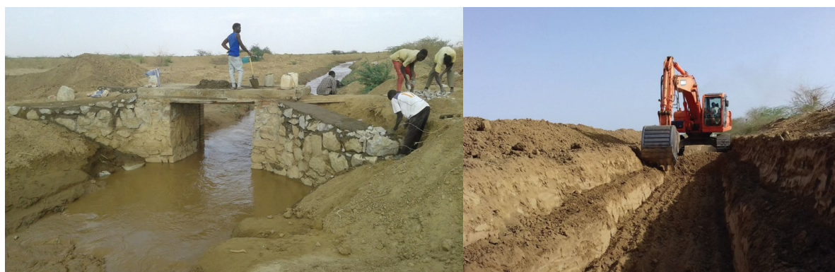
Figure 2-4: Low-cost intake and field canals that contributed to improved field water management and productivity in Gash seasonal river based agricultural scheme in Sudan (Credit: Amira Mekawi, HRC)
